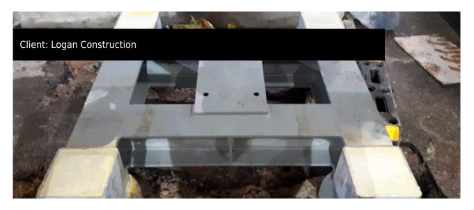
ScrewFast were chosen by main contractors Logan Construction to design, build and install the foundations for a MRI Gantry Supports at the Royal Free Hospital in Hampstead, London.
