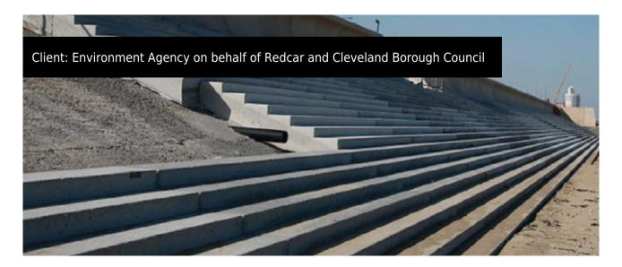
The Environment Agency awarded a £21M contract to Birse Coastal, a Birse Civils company, to construct a scheme at Redcar to minimise the risk of coastal flooding to more than 1,000 properties. The new defences stretching for 2.7 kilometres and are intended to reduce coastal erosion and flood risk for the next 50 years and beyond.
