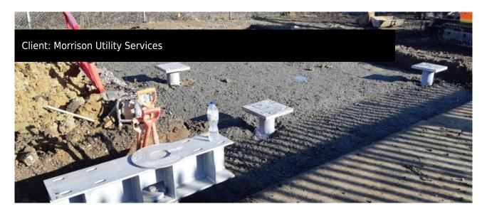
As part of ScrewFast Foundations long-standing relationship with Morrisons Utilities, we were contracted to install foundations at two further locations. The ScrewFast design team recommend helical pile foundations at the majority of substation sites because the installation process requires minimal plant and no excavation. This significantly reduces risk involved with the foundations process with the proximity to overhead high voltage cables, as well as underground cables and services.
