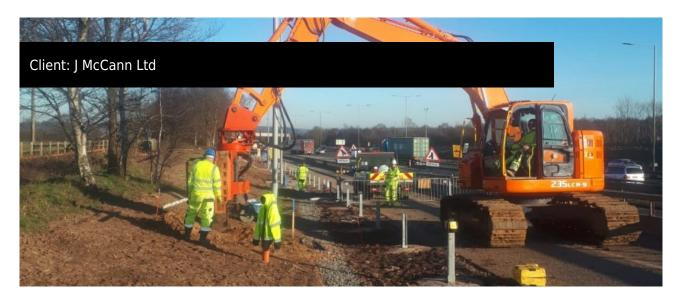
ScrewFast Foundations were contracted by McCann Ltd to design and install foundations for new Fixed Vertical Road Traffic Signs on the M6 Motorway between Junctions 2 and 4.
