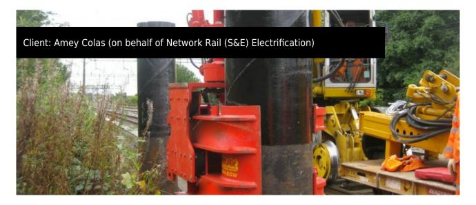
The client sought a solution to support 2 Twin Track Cantilever (TTC) Overhead Line Electrification(OLE) structures and 2 Anchor Masts each with a Tieback Anchor.
